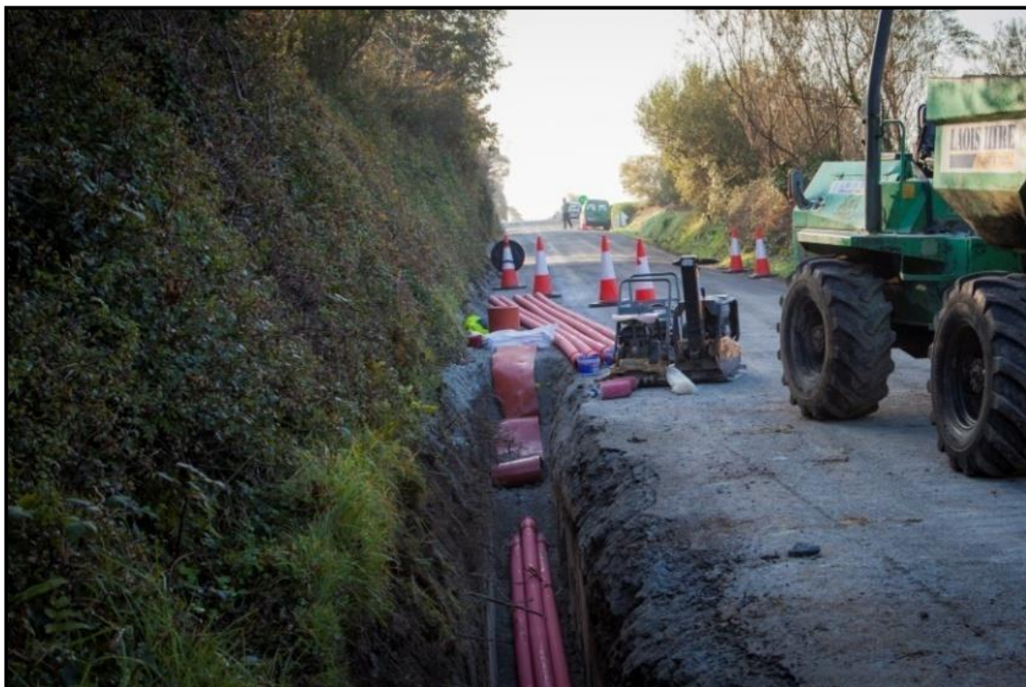
Figure 3-18 Typical ducting installation works for a grid connection cable trench
