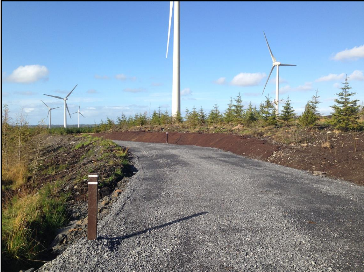
Figure 3-13 Typical new excavated road on a wind farm
