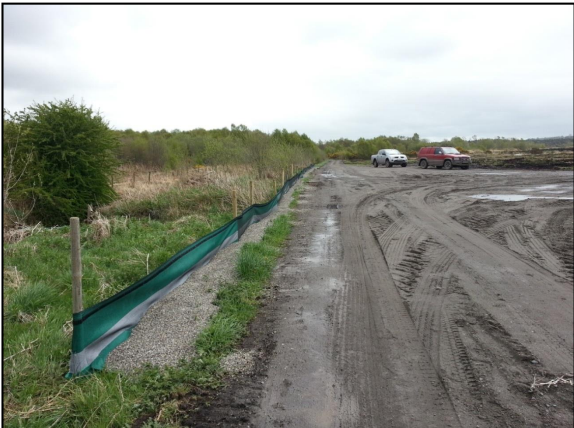
Figure 3-31 Silt curtain containment along existing roads near watercourses
