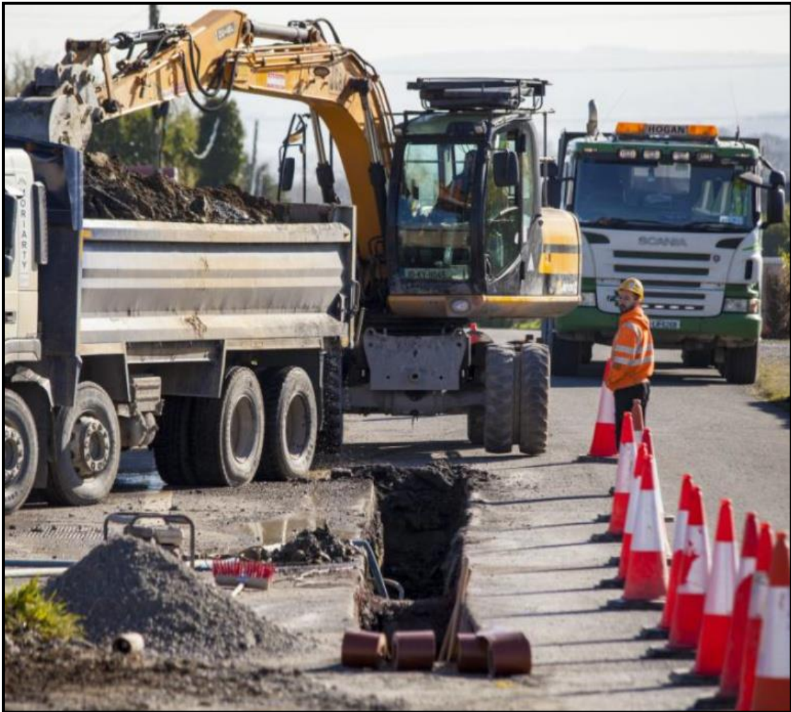
Figure 3-17 Typical excavation works for a grid connection cable trench
