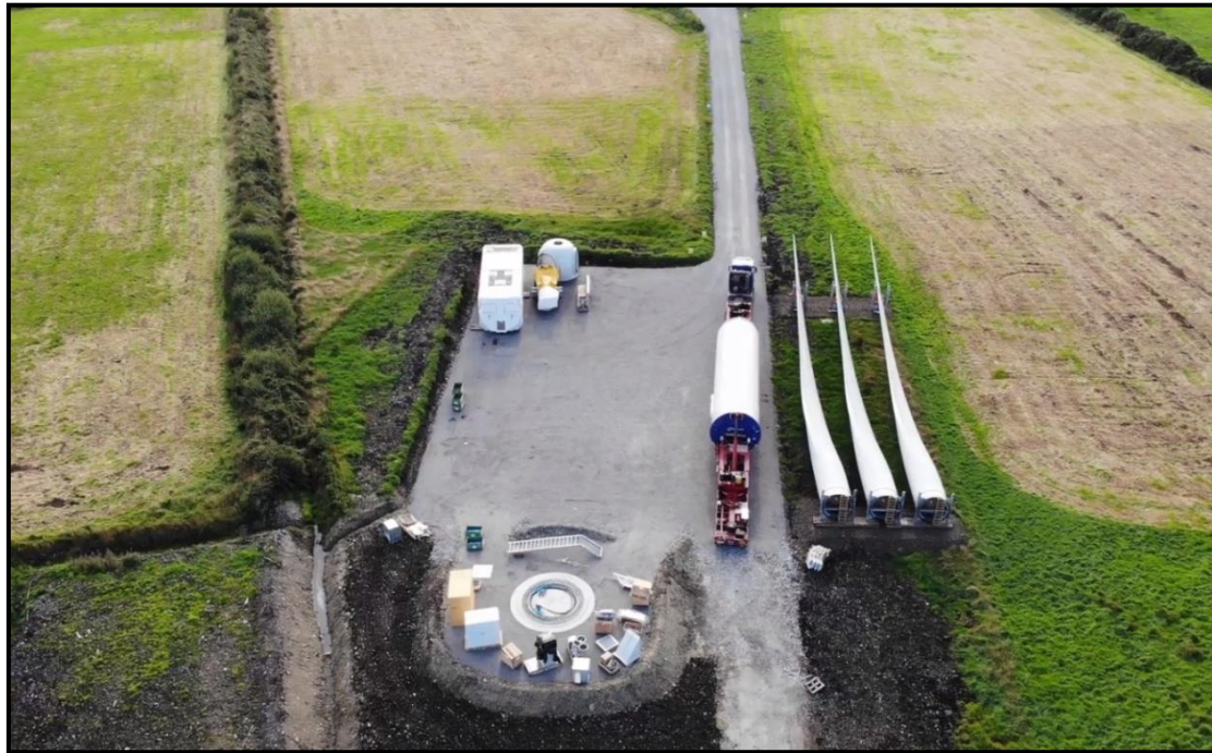
Figure 3-15 Typical finished hardstand on a wind farm
