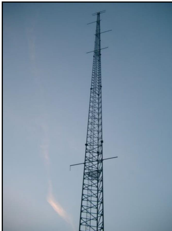
Figure 3-23 Typical meteorological mast on a wind farm
