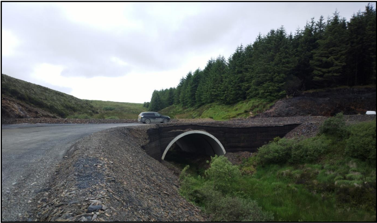
Figure 3-28 Completed clear span pre-cast concrete culvert crossing over existing watercourse
