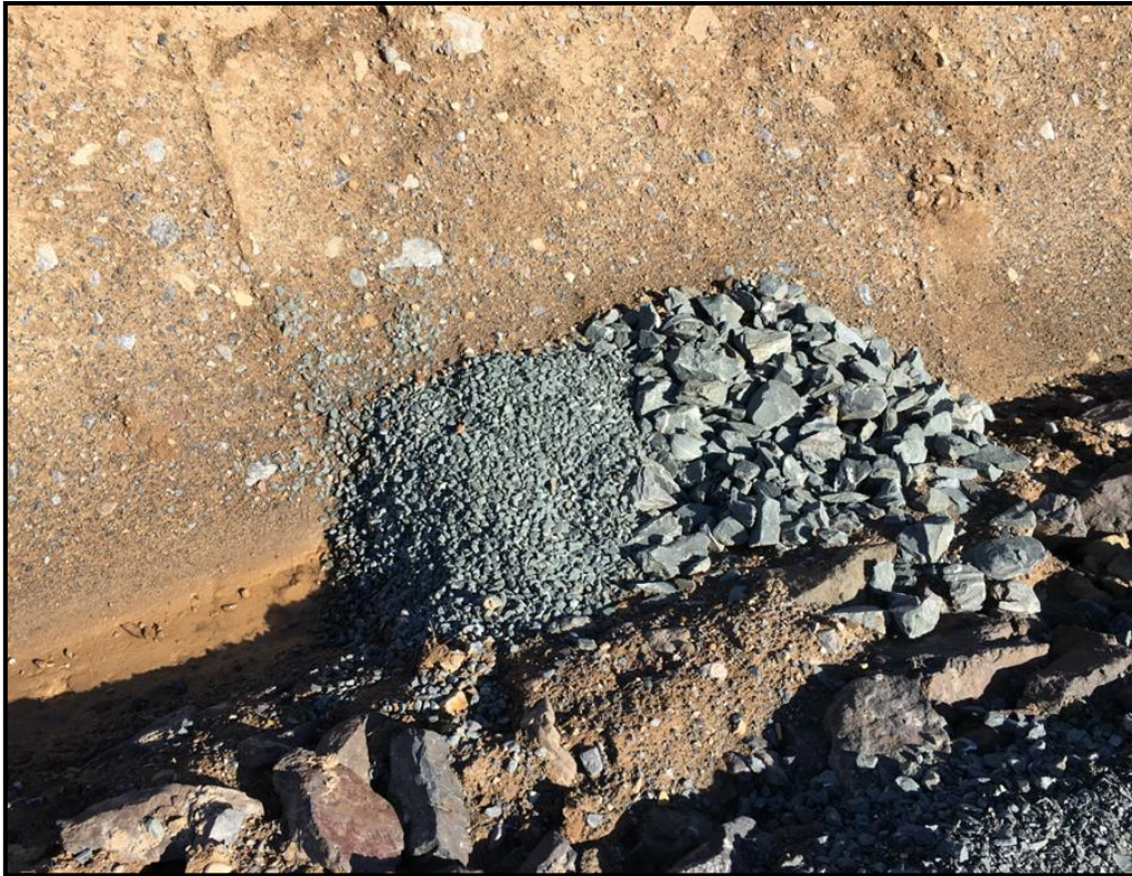
Figure 3-32 Stone check dam with large aggregate on downstream side
