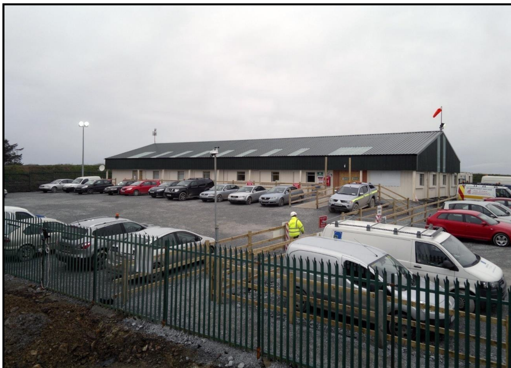
Figure 3-25 Typical temporary site construction compound on a wind farm
