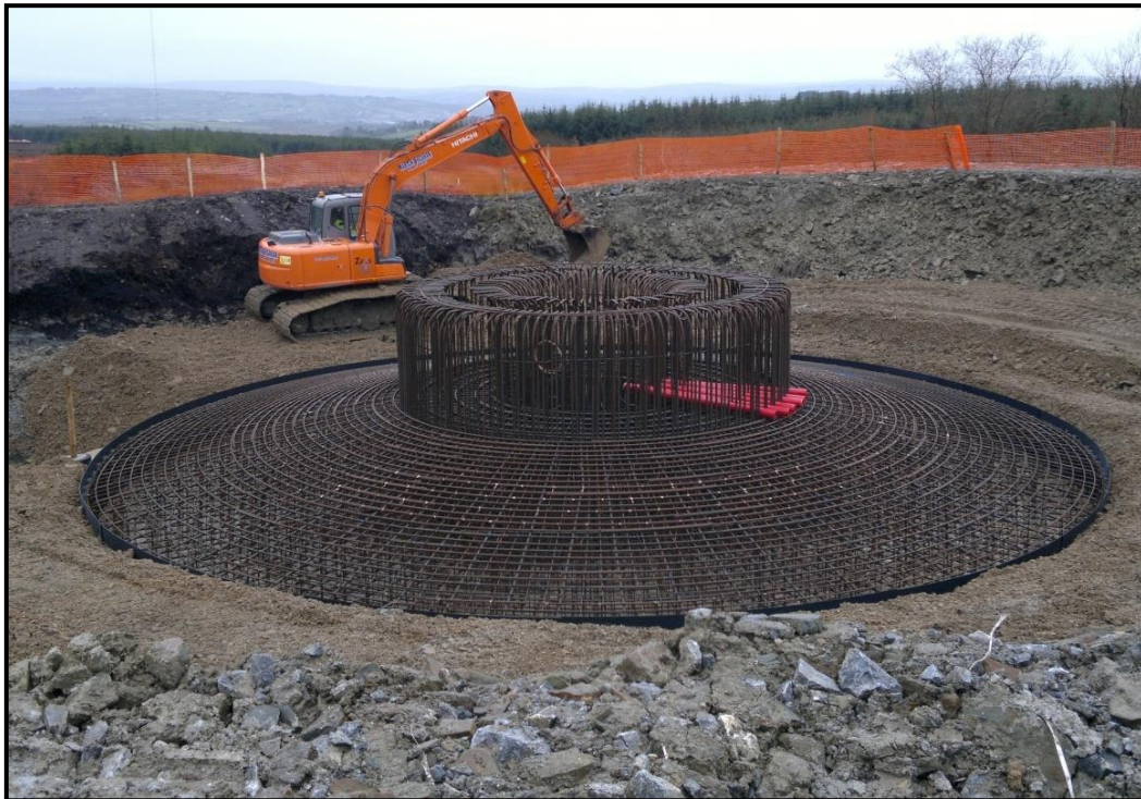
Figure 3-16 Typical construction of a wind turbine base
