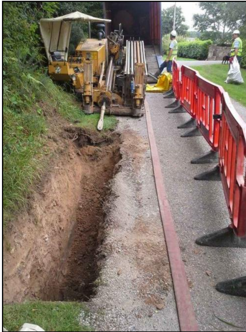
Figure 3-20 Typical directional drilling rig and launch pit
