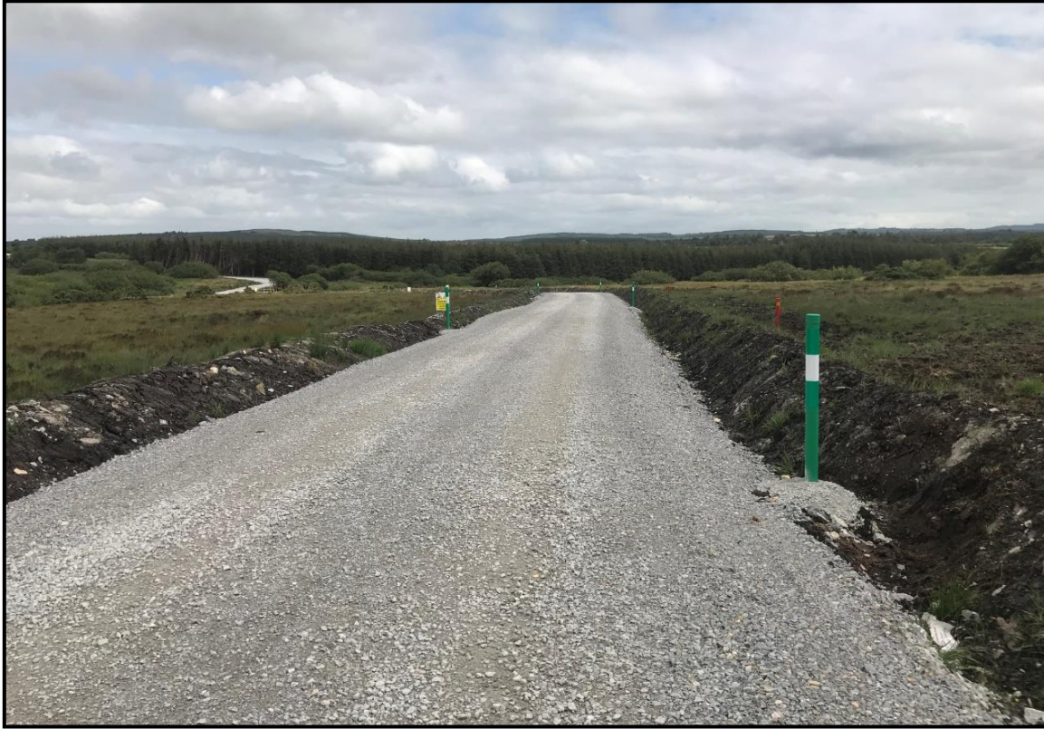
Figure 3-14 Typical floated road on a wind farm
