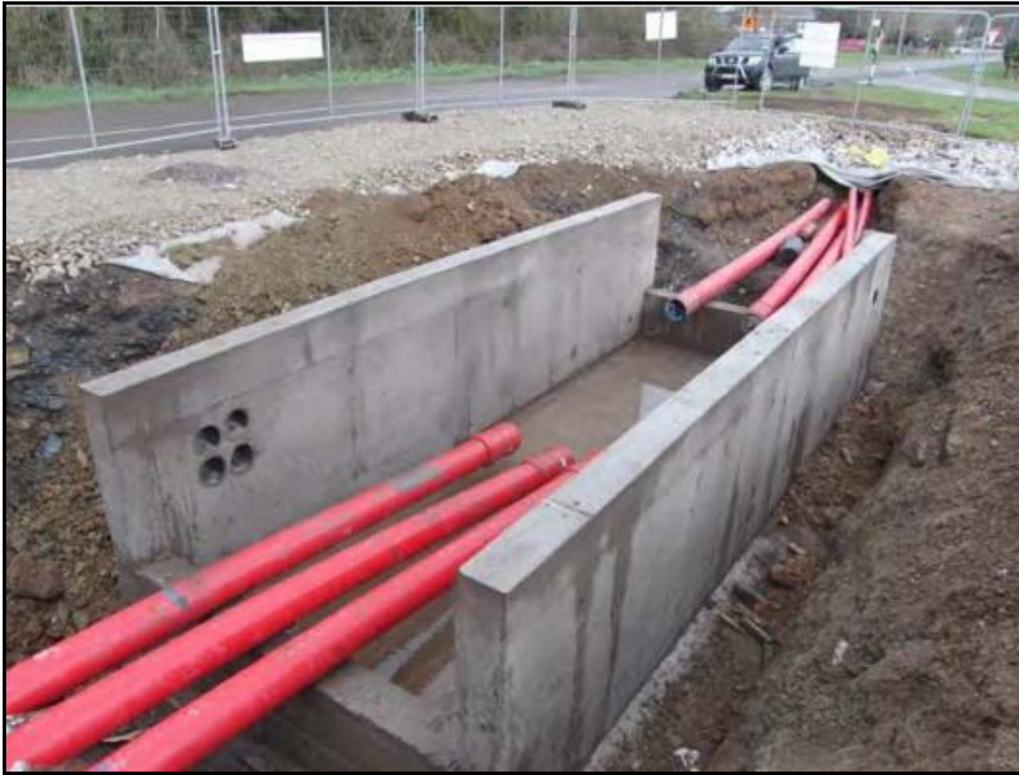
Figure 3-21 Typical joint bay construction
