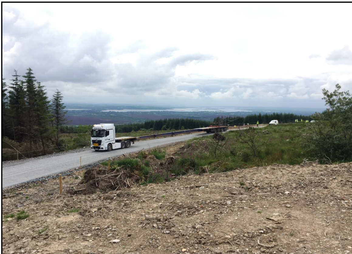
Figure 3-12 Typical upgraded forestry road on a wind farm
