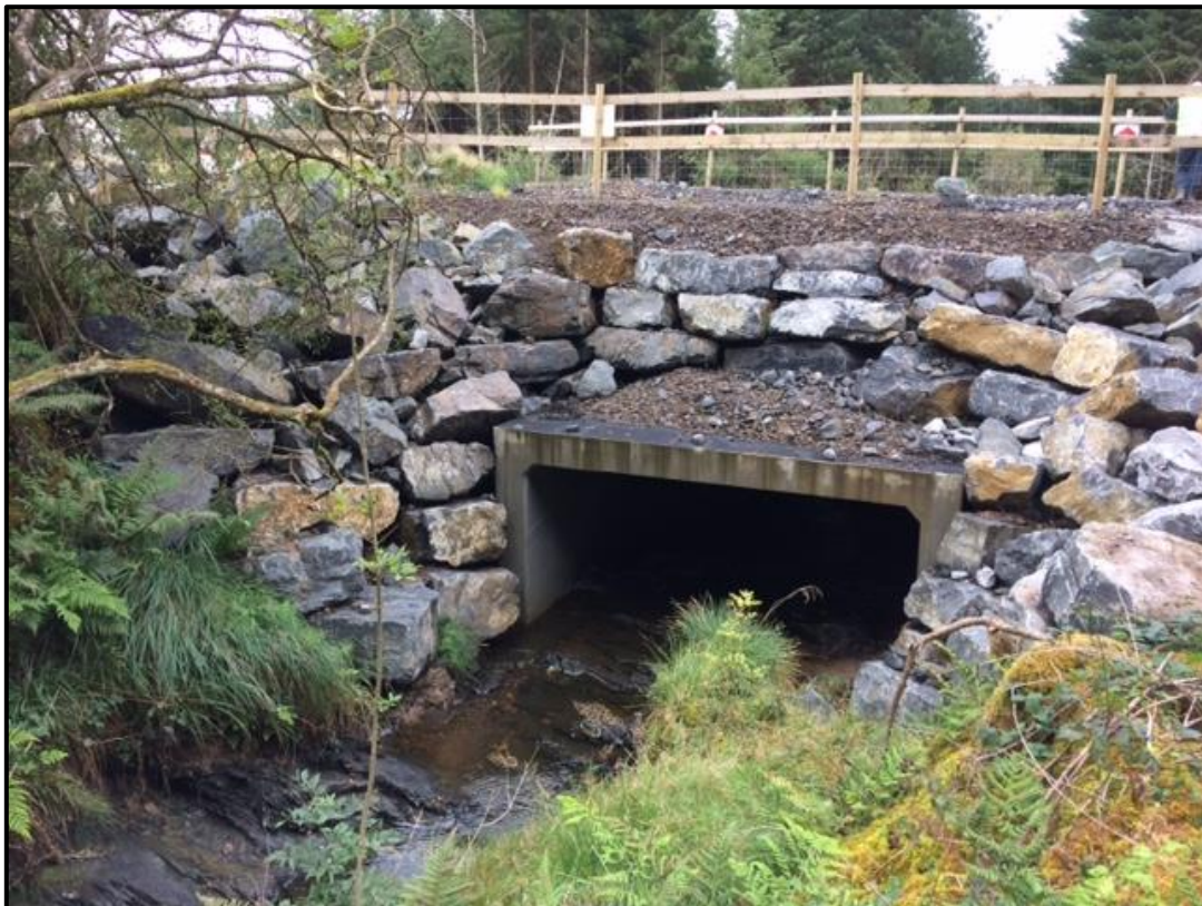
Figure 3-29 Typical drainage channel crossing
